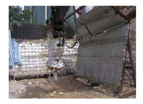
The acoustic wrapping for the percussion breakers of excavators and the noise barrier comprise of minimum 50mm thick sound absorbing lining with a hard backing plate for the noise barrier.
